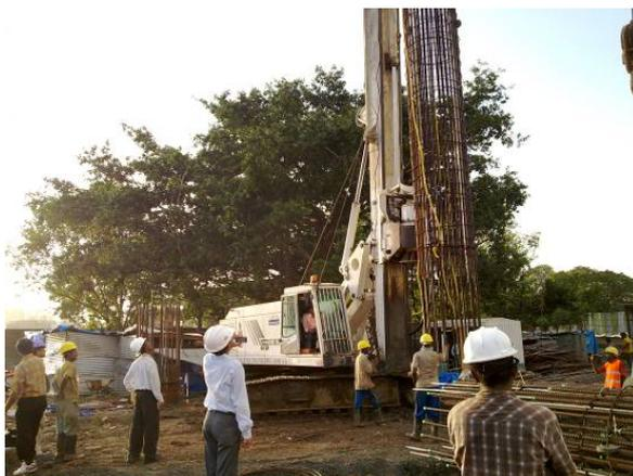
Hoisting and Installation of Cages
