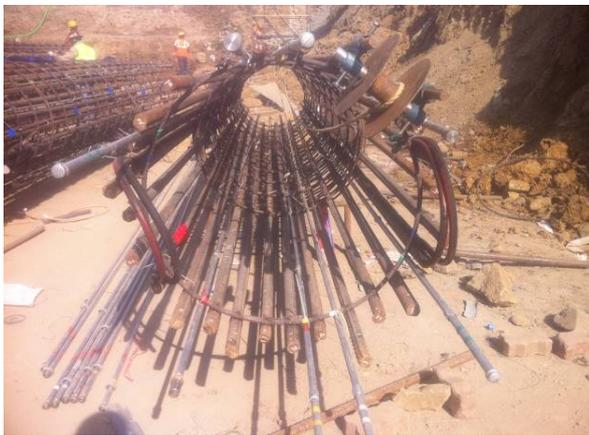
Instrumented Cages Ready For Installation
